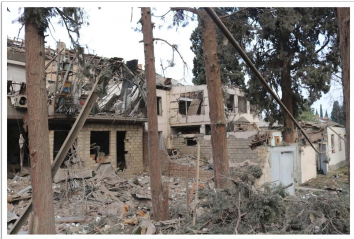
Photo 3-4: Destroyed residential buildings, Ganja, Azerbaijan
