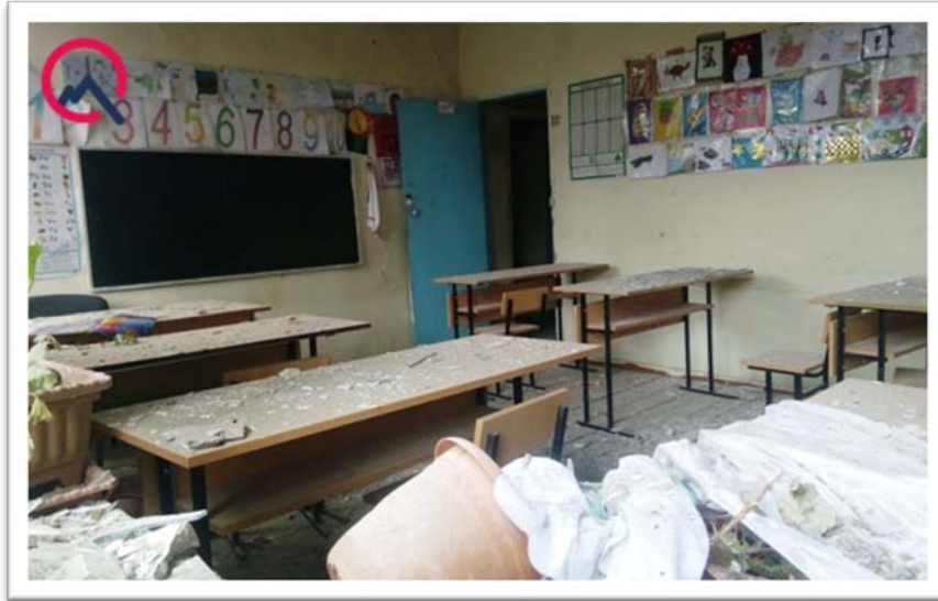
School building in Terter district damaged by artillery shelling:
