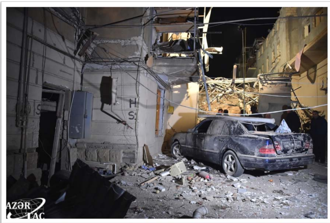
Photo 5-6: Destroyed residential buildings, Ganja, Azerbaijan
